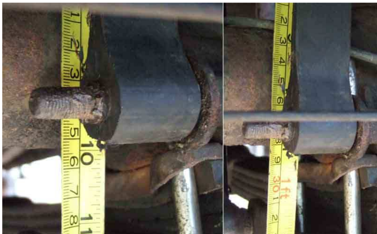
Clear signs of reinforcing in the original (top), none in the current stock
