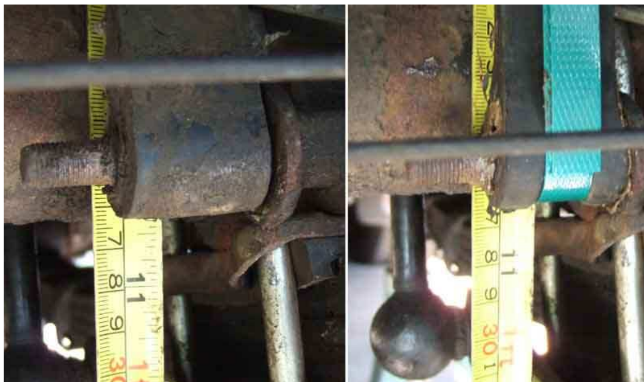
Fully fitted, with cable tie
