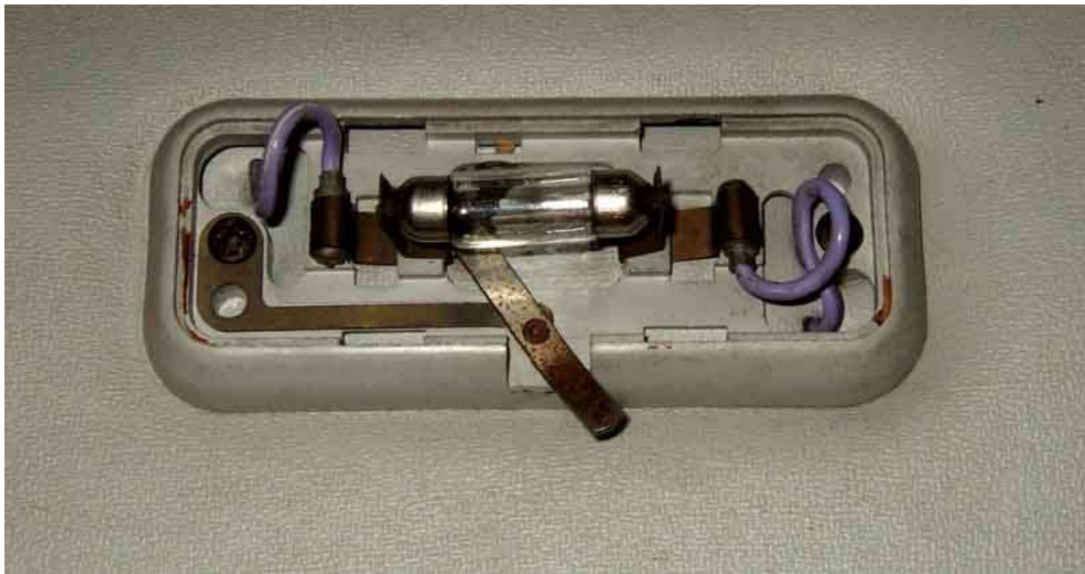
The manual switch (arrowed), depressed by the tab on the hatch to turn the light off.
