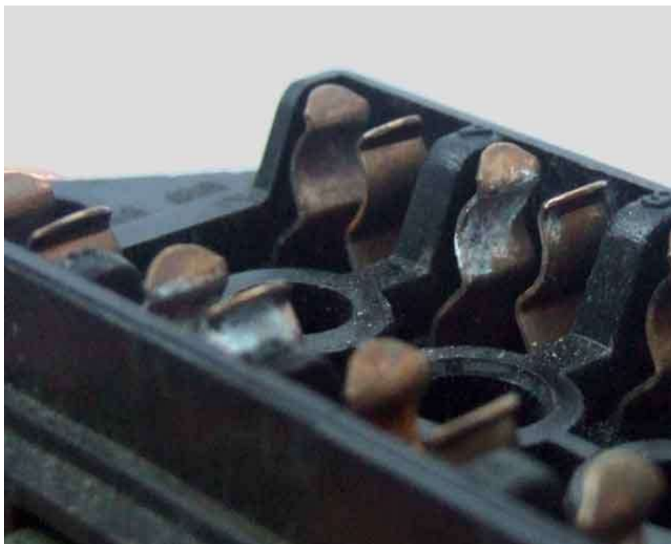
Fusebox cover with spare fuses.
