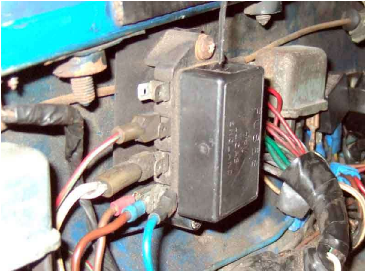
... is an insulating sheet between the fusebox and the spacers. 3/16" UNF screws (note the lower one is sheared) into welded nuts on the back of the inner wing.
